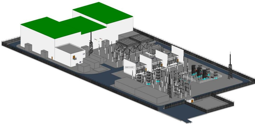
**Figure 4 Converter Station Alternative Configuration 1 3-D View** (source: WSP | not to scale)
