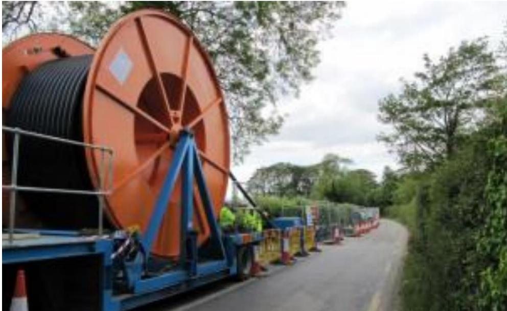
**Figure 9: Cable Drum at Joint-bay location**
