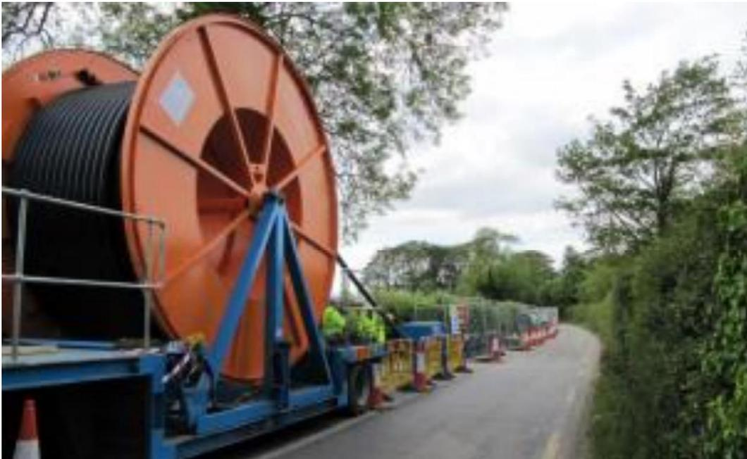
**Figure 4.13: Cable Drum at Joint-bay location**
